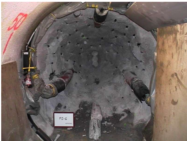
CONCRETE PLUG DEMOLITION
