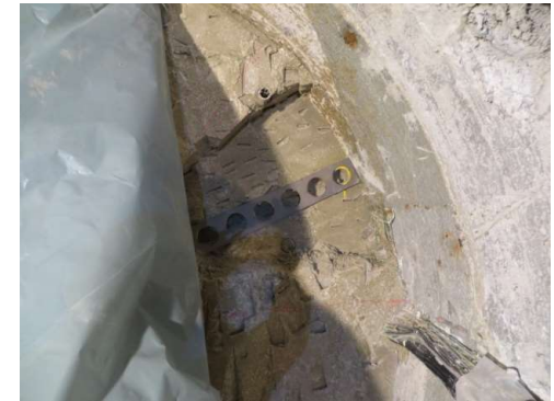
Drilling following a template
