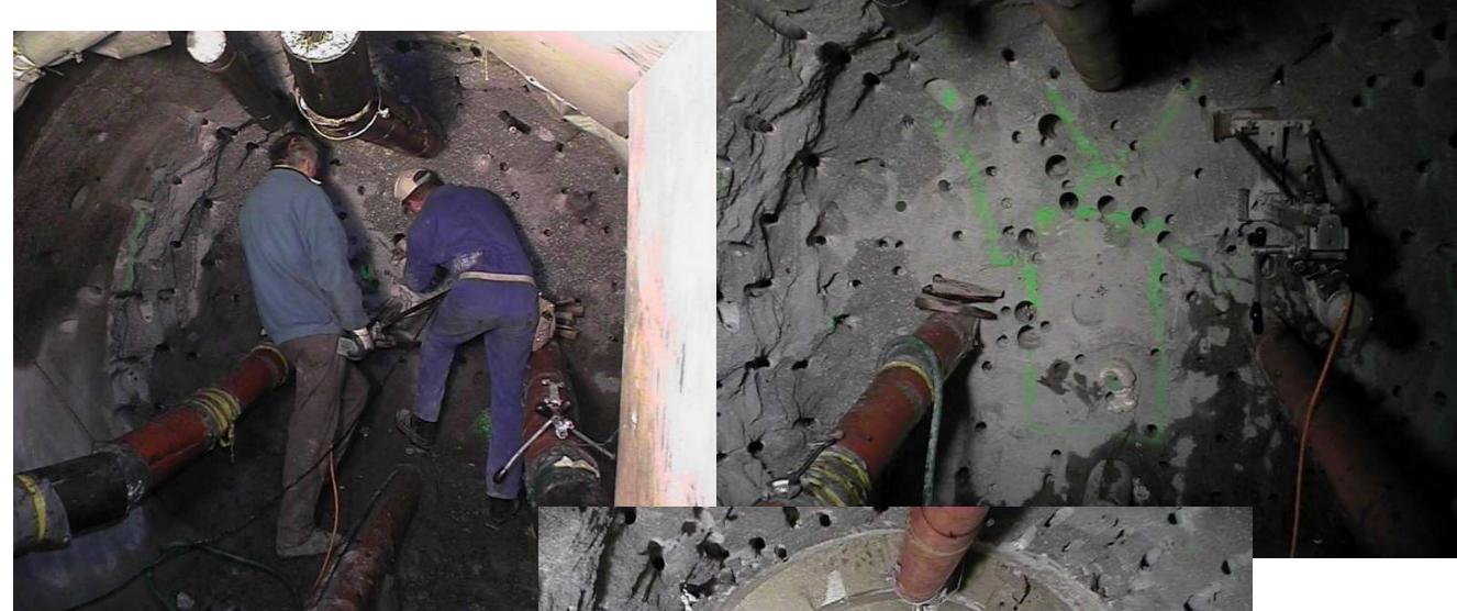
CONCRETE PLUG DEMOLITION
